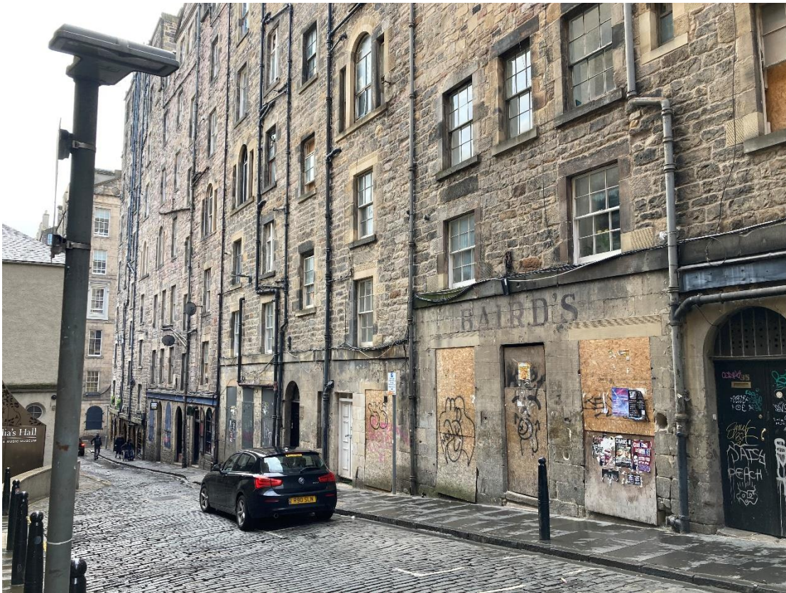
Figure 16 - Niddy Street to south of access
