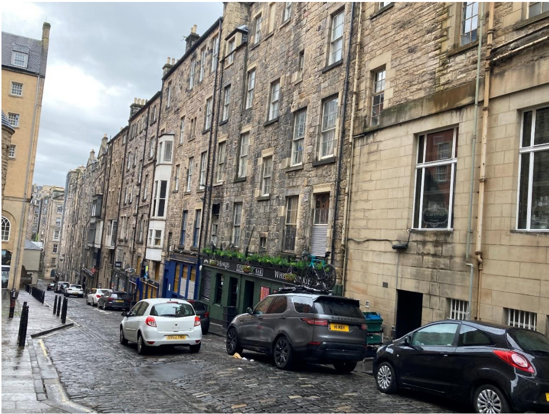
Figure 6 - View south, down Niddry street, opposite side
